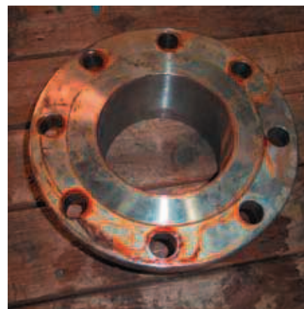
Fig. 5. RVS 304 flange contaminated by ferruginous water.
