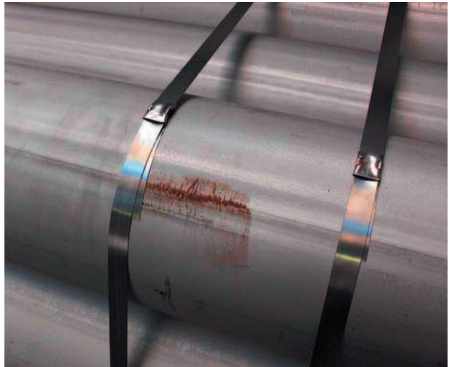
Fig. 3. Contamination by a steel object such as the fork of a forklift truck.
